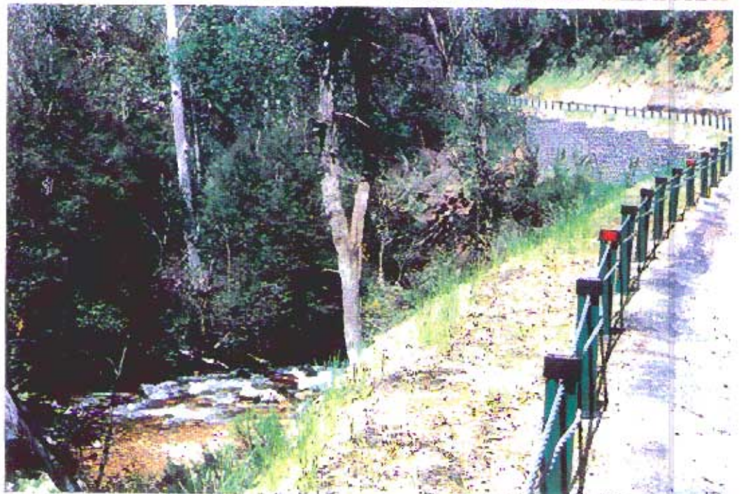
Another view of Leatherbarrel Creek on the Alpine Way, the site of recent major reconstruction works. One of the main considerations in choosing Briten WRSF was its low visual impact on the landscape.
