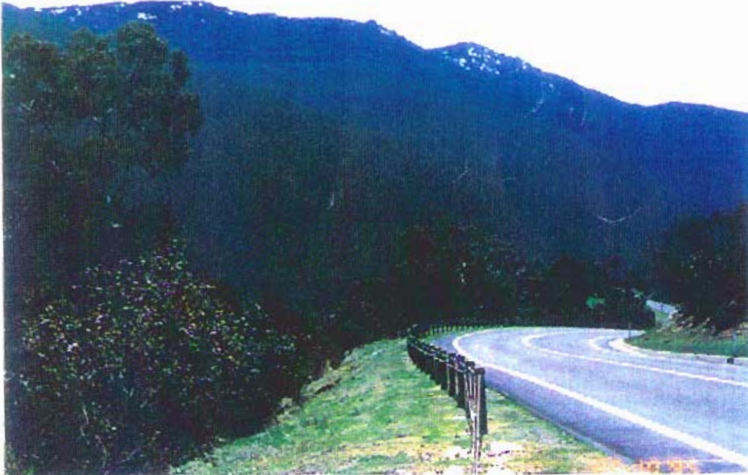
Another aspect of Alpine Way near Thredbo where visitor-use is high all-year-round. Here too, Brifen WRSF provides protection for motorists whilst having minimal impact on the views of Thredbo Valley.
